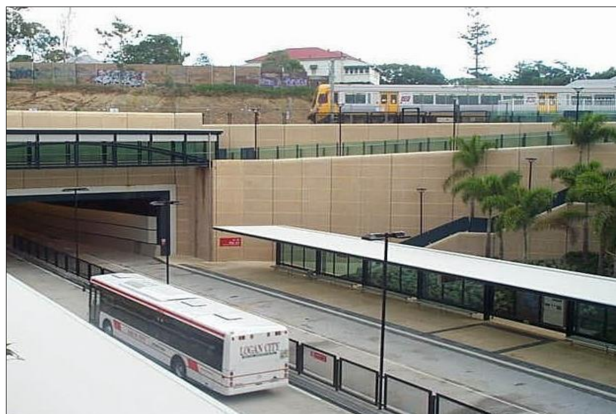
Example of a BRT System
